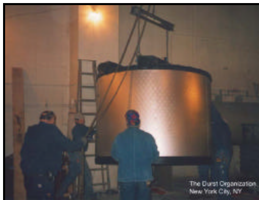
Rigging C-Model Icebank into place.
