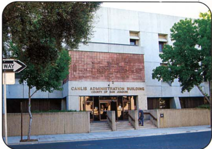
While a chiller retrofit helped save money in the Canlis Administrative Building (Stockton, CA), San Joaquin County energy manager David LaLonde estimates that the new ice TES system saves an additional $3,000 during an average summer month.
