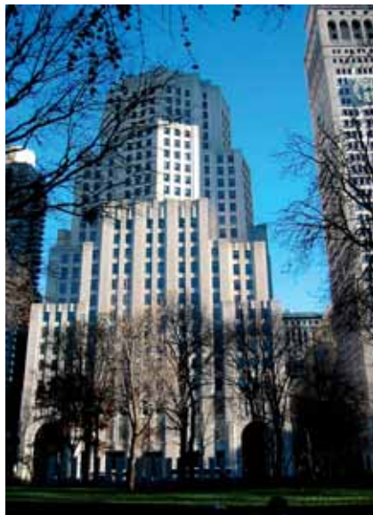
Energy-efficient replacement chillers from Trane and an ice storage system from CALMAC enable this 2.2 million-square-foot office building, which houses the national headquarters of Credit Suisse, to save 2,153,200 kWh per year and lower peak energy usage by more than 900kW, according to NYSERDA.
