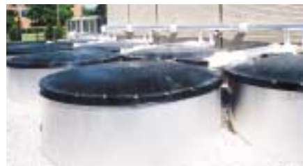
Fairfield Elementary School, Fort Wayne, IN
