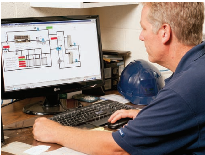
A building automation system provides building control through a single, integrated system, while energy storage tanks provide cooling.
