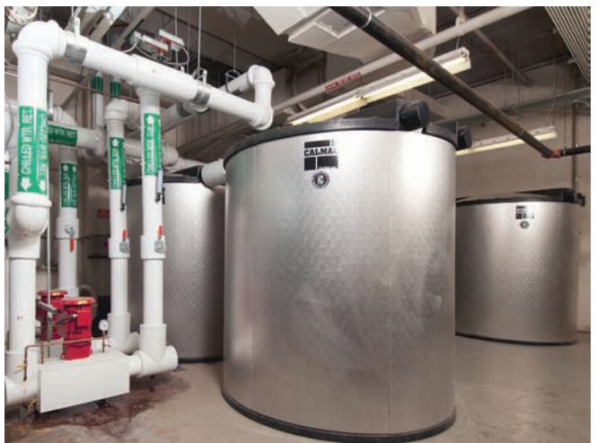
A building automation system provides building control through a single, integrated system, while energy storage tanks provide cooling.
